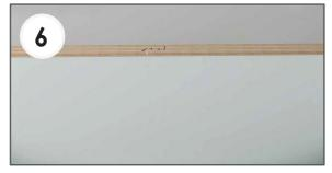
Remove the masking tape and ensure any excess silicone adhesive is wiped from the laminate face immediately.
