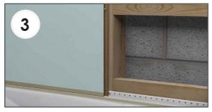
Fix through the back flange of the grooved edge with countersunk screws - the screw head should fit into the recess on the back of the tongue. Ensure that screws are turned until they are just under the flush to prevent any obstruction to the tongue of the next panel to be fitted.
